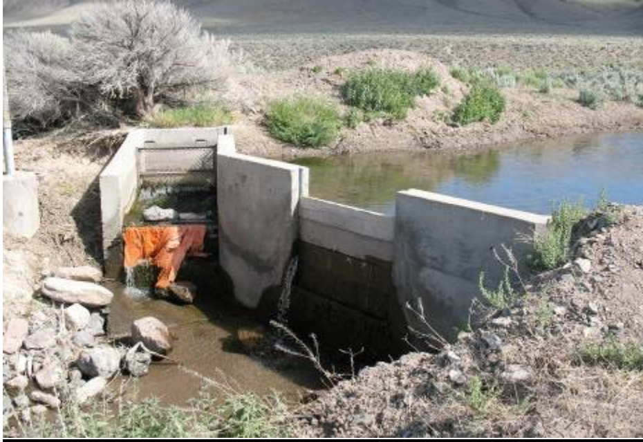
Photo 1. Water diversion into pipeline (May 2007).
